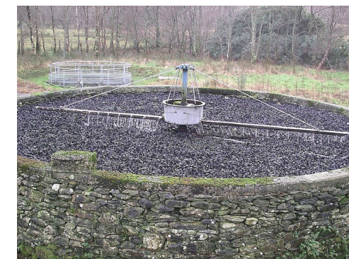
Realisation of a trickling filter
