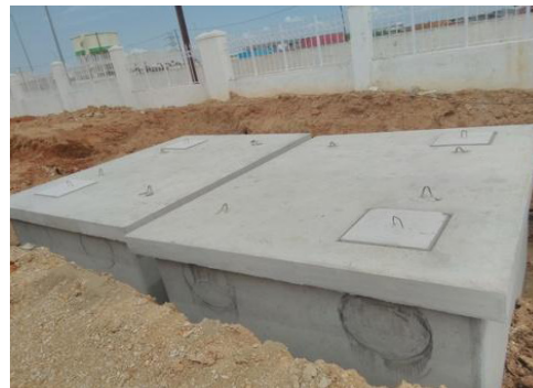
Settler tank under construction
