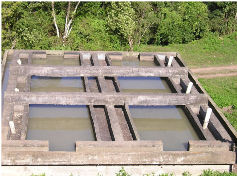
Imhoff tank without grating
