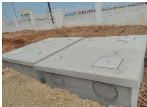
Settler tank under construction
