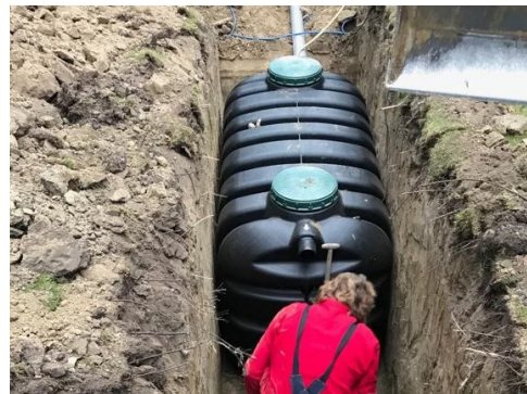
Underground septic tank
