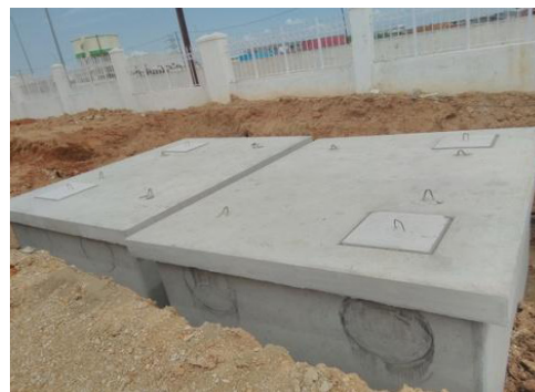
Settler tank under construction
