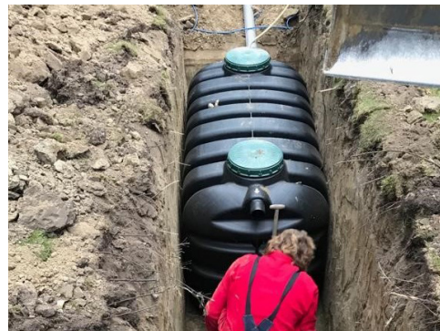
Underground septic tank
