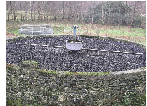
Realisation of a trickling filter
