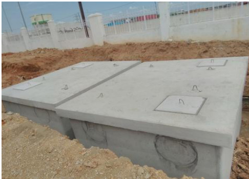
Settler tank under construction
