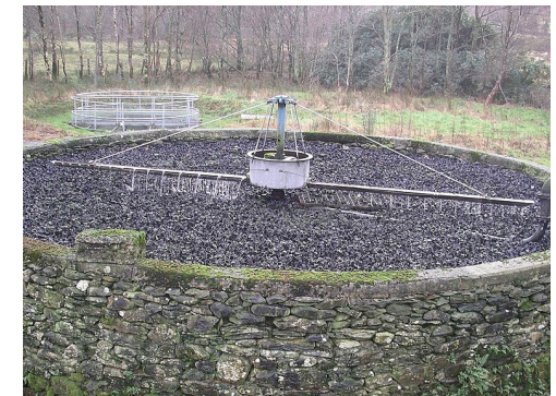
Realisation of a trickling filter
