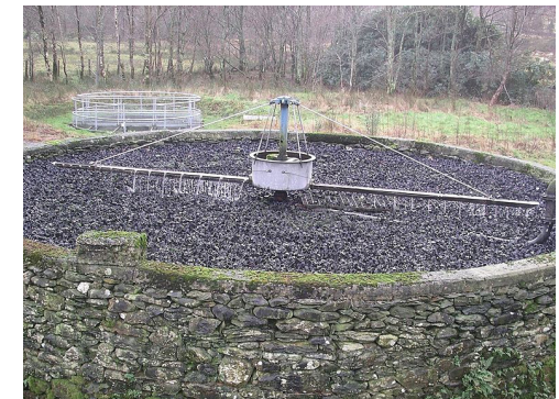
Realisation of a trickling filter
